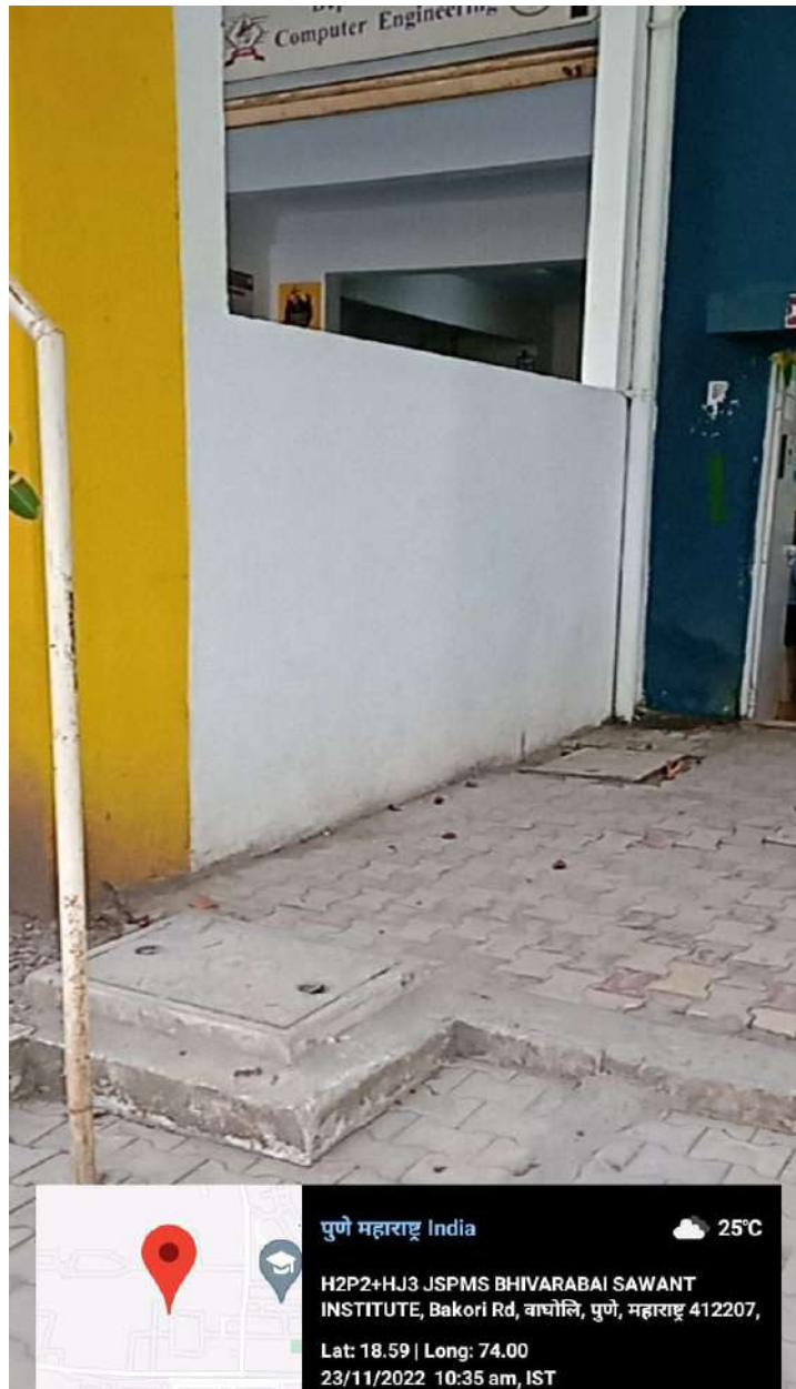
Fig. 5 Rain water storage
