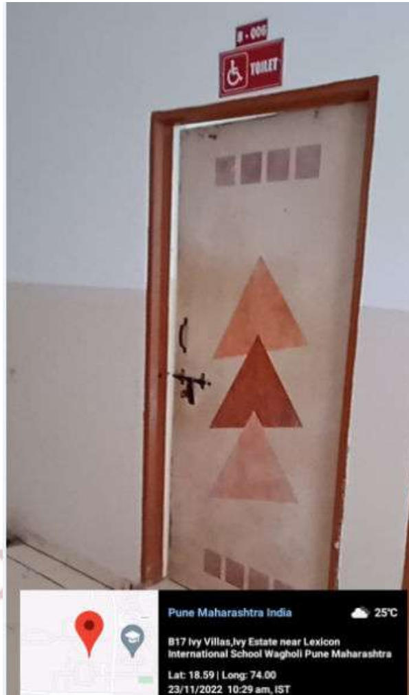
Fig. 12 Toilet for disabled of ICOER
