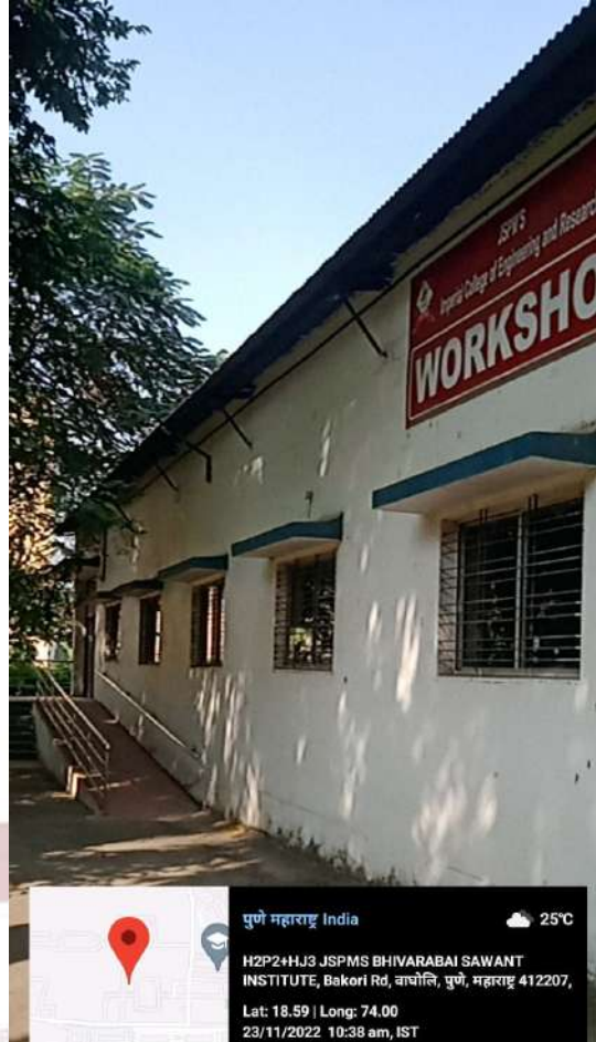
Fig 11 Ramp at central workshop of ICOER
